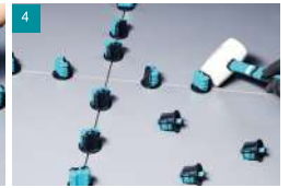
4 Remove the cap with BI-HUI rubber mallet and open the cap simply for reuse
