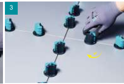
3 Close the cap and spin down to the required level to ensure no lippage
